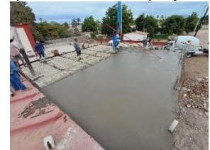
Pouring roof in January
