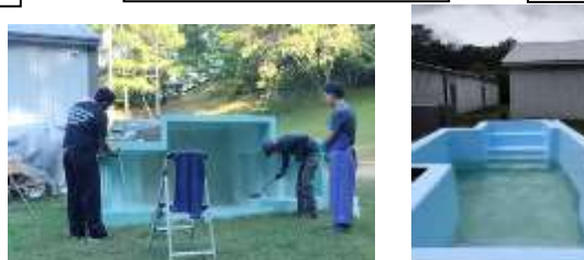
Preparing the baptistry
